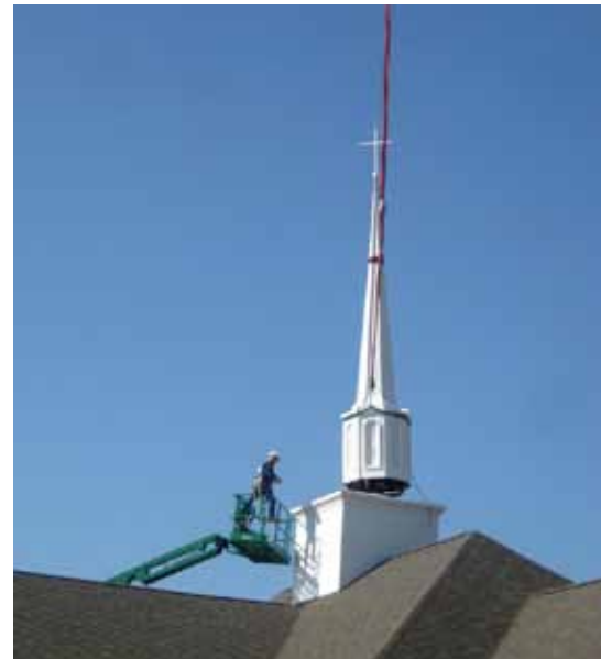
The steeple is lowered into place on the new Christ Lutheran-Perry building.
