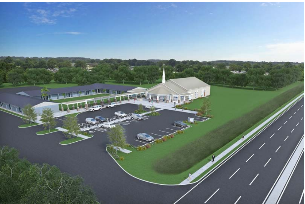
Hope/Plant City, FL's new sanctuary will seat 300 compared to the current 190 with ample room for the congregation's music and other worship ministries. This is phase one of a three-phase building program for Hope. The additional phases will relocate their offices allowing additional space for fellowship events and provide a larger kitchen area. Hope's current sanctuary will be demolished following completion of the new building to allow room for handicapped and visitor parking along with a covered walkway connecting Hope's campus. Hope began serving the Plant City community in February, 1957. Two of Hope's initial founding five families, continue to be active in the congregation. Projected completion date of the new facility is Spring of 2021.
